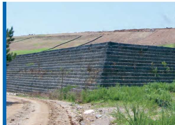
Figure 2. Stratagrid and backfill used along with wire baskets.
