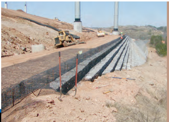
Figure 1. Wire baskets are used for the facing of the
