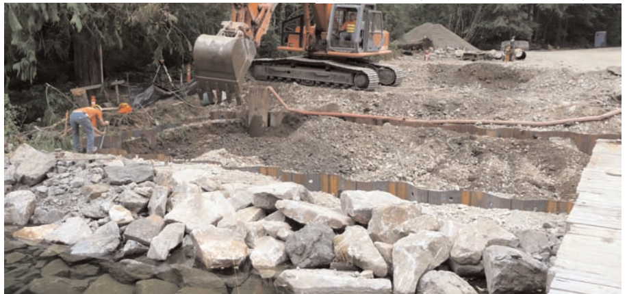
Excavation for the new bridge abutment.
