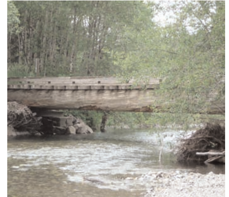
Original timber bridge supported by timber cribbing.
