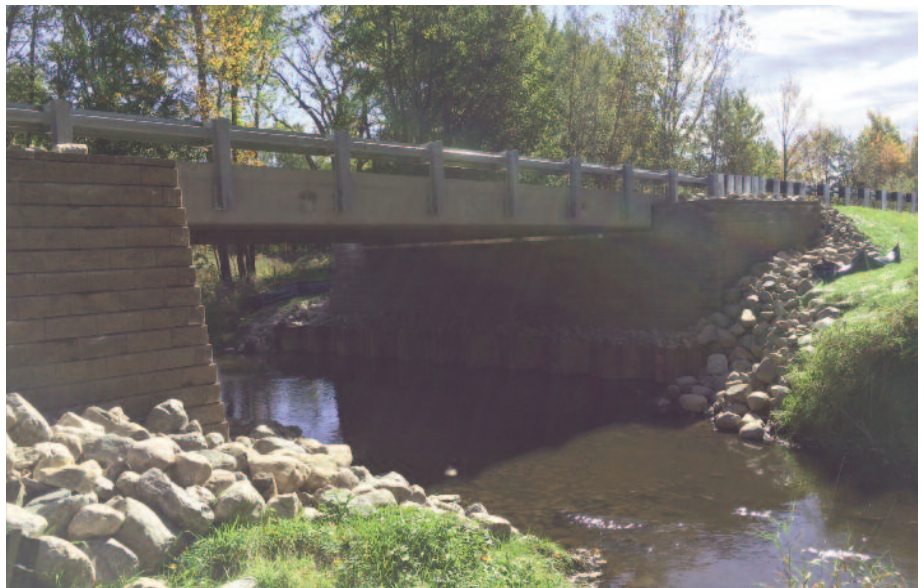
Completed Keefer Highway Bridge abutment ready for traffic.
