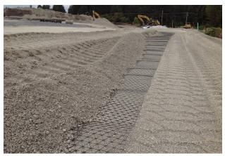
Tensar® TriAx® Geogrid was installed to help resolve soil stabilization challenges over the capped landfill.
