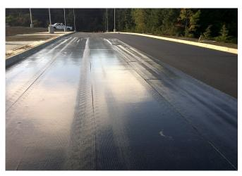
GlasGrid TF with pre-installed tack film was installed in the bus and traffic areas to reinforce the pavement.
