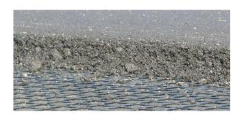
GlasGrid Pavement Reinforcement System
