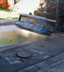
With proper design and placement, interlayers can add traffic capacity to the aslphalt pavement.
