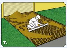
Fill Turf Cell<sup>®</sup> grass pavers with a mixture of sand & topsoil (growing Media) or compost
