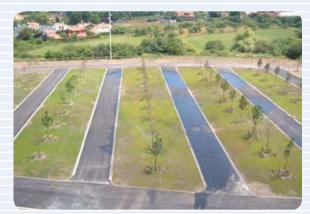
Gravel Cell® reinforcement structure used for access roads. Turf Cell® reinforcement structure used for parking bays.
