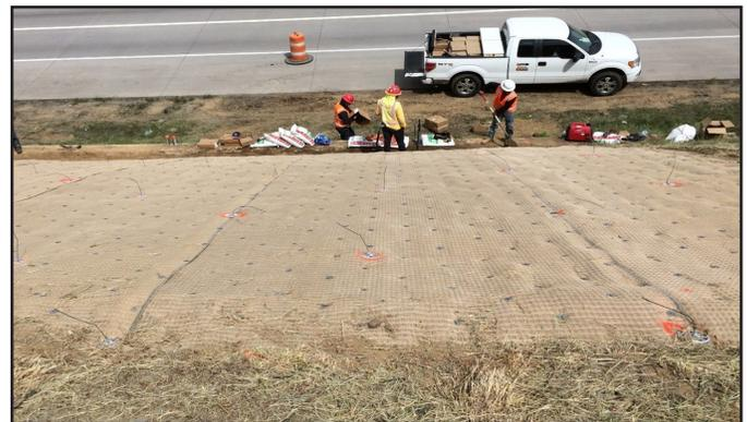
*Rapid snow melt and spring rains resulted in shallow slope failures (top). The XAS system installed with percussion driven anchors over prepped and seeded soil, provided surficial slope stability and resulted in a stable vegetated slope (center, bottom).*
