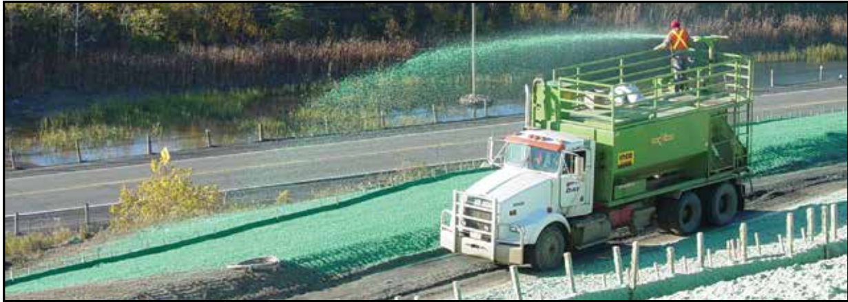
Sodium-pHix can be applied using a hydraulic seeder to help lower the salinity and increase the level of calcium in the soil.
